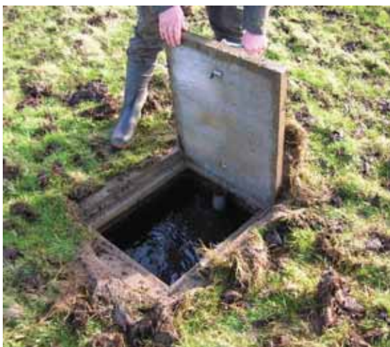
John Gerrard inspecting a sub-surface pipe sluices (left) and soil bund and pipe sluice backing water up one of the existing ditches © Gavin Thomas (RSPB)
