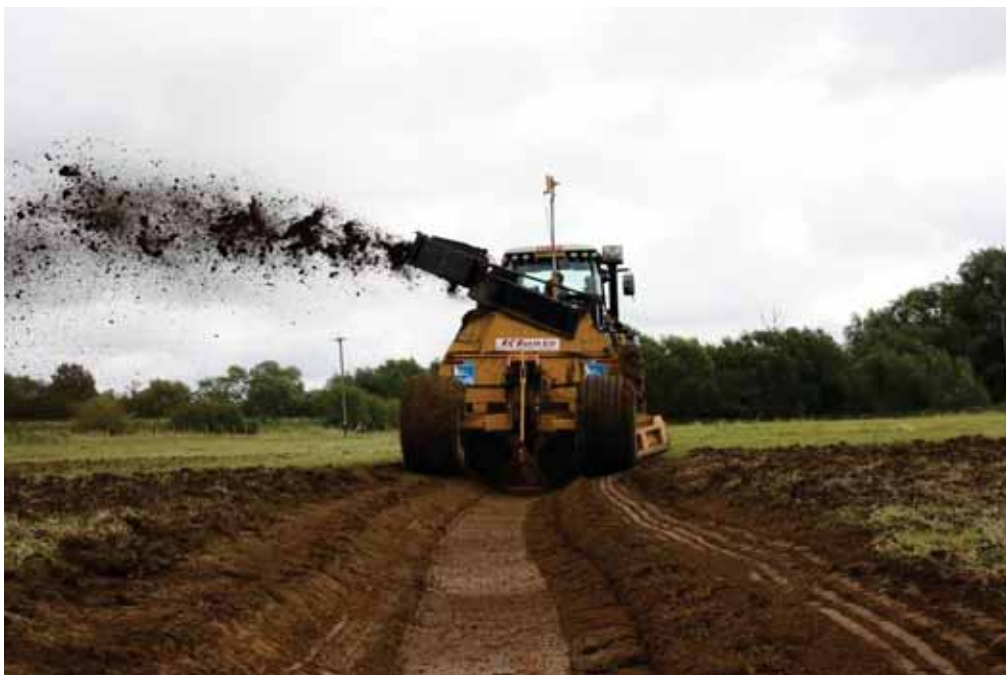
Creating a foot drain at Chimney Meadows Nature Reserve © Mike Shurmer (RSPB)
