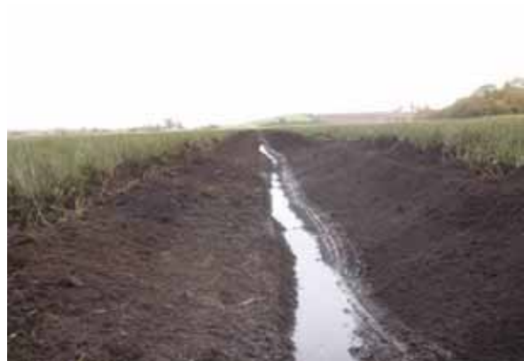
The BOS spoil spreader and SoucyTrack on a wet peat site and a foot drain created with this set up © RC Baker Ltd.
