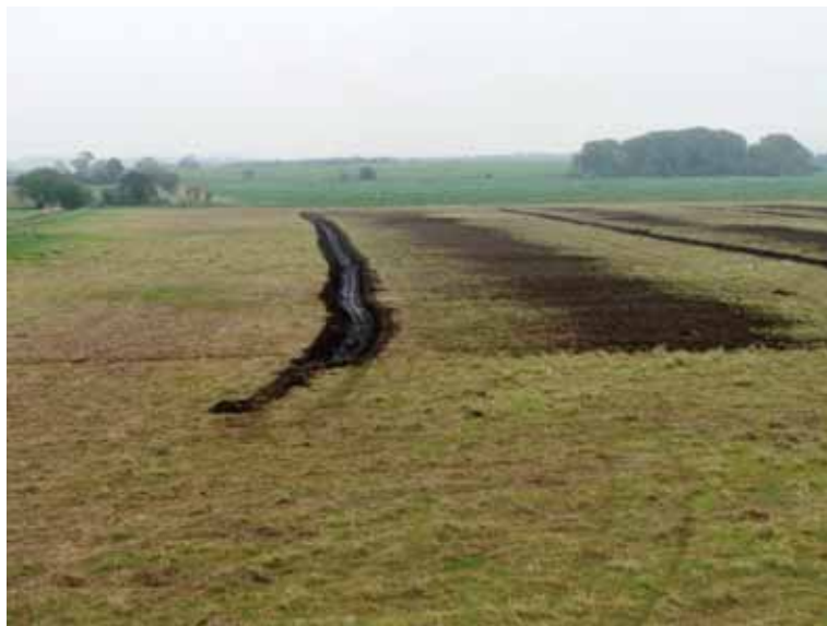
Spacing foot drains on a peat site © Natural England
