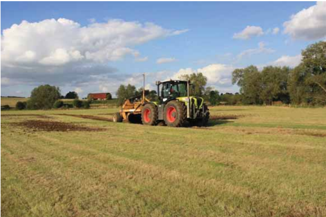
The rotary ditcher at work © Mike Shurmer (RSPB)
