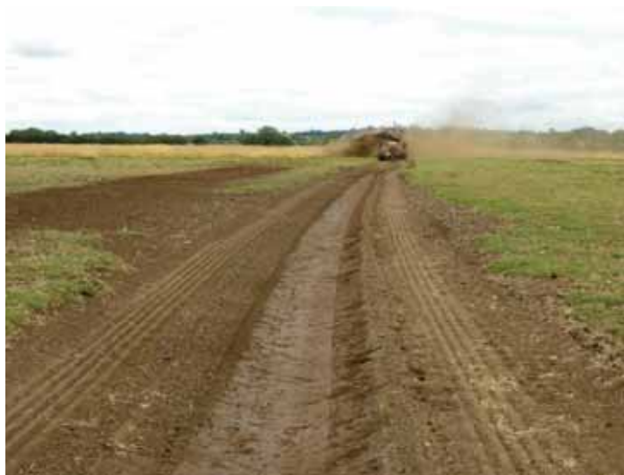
A freshly excavated foot drain on the Cherwell © Mike Shurmer (RSPB)
