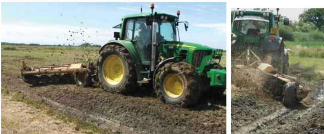
Cleaning out an existing foot drain © RSPB
