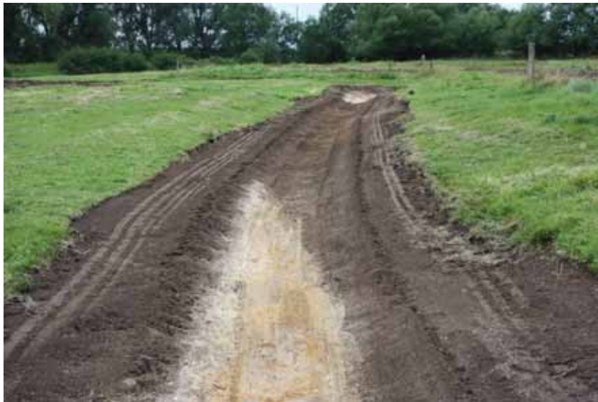
Check soils to avoid situations like this foot drain breaking the gravel layer © Mike Shurmer (RSPB)
