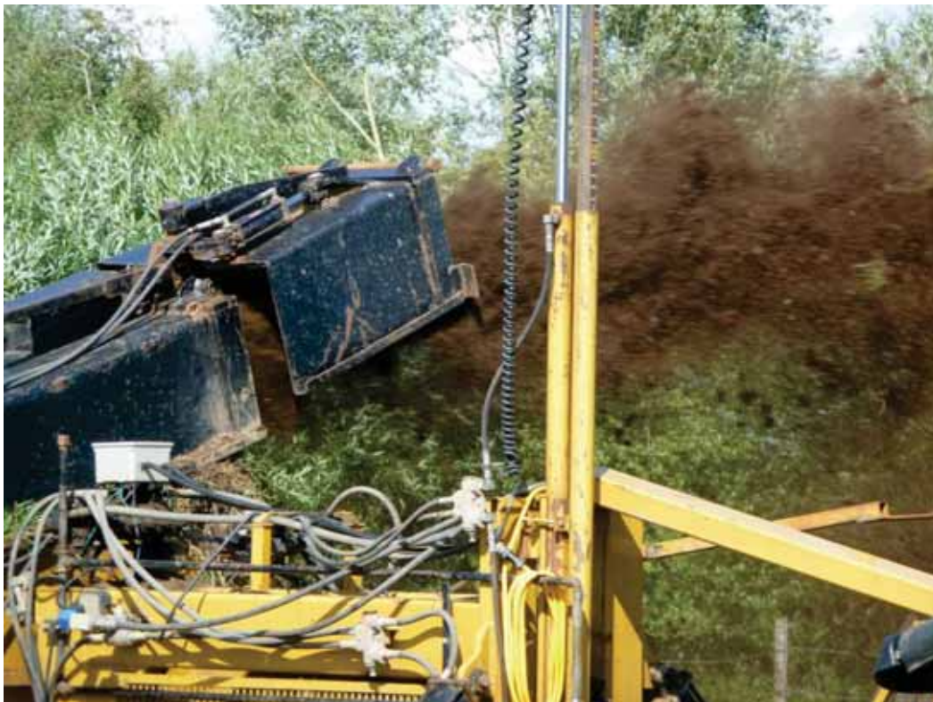
Spreading spoil © RC Baker Ltd.
