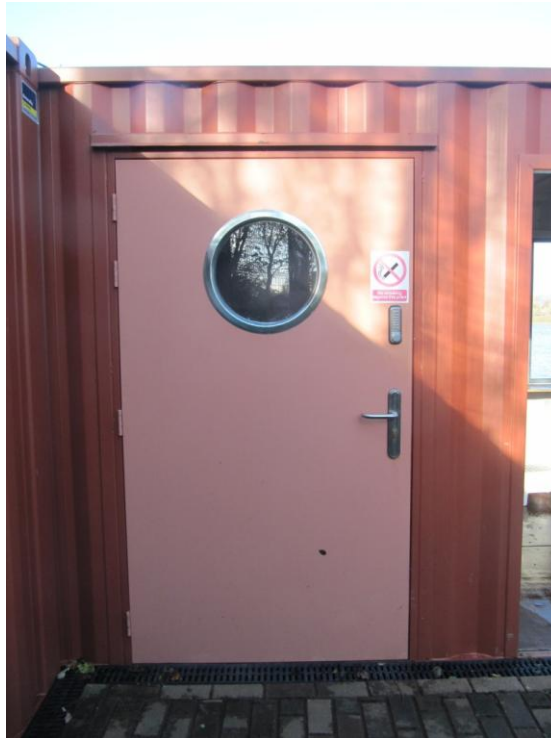
Figure 4 The members area is accessed by a code pad, 145cm from ground level.
