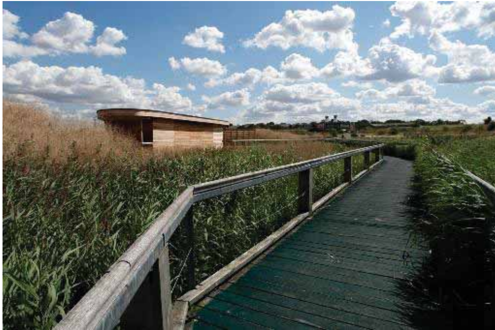
A section of boardwalk on the reserve
