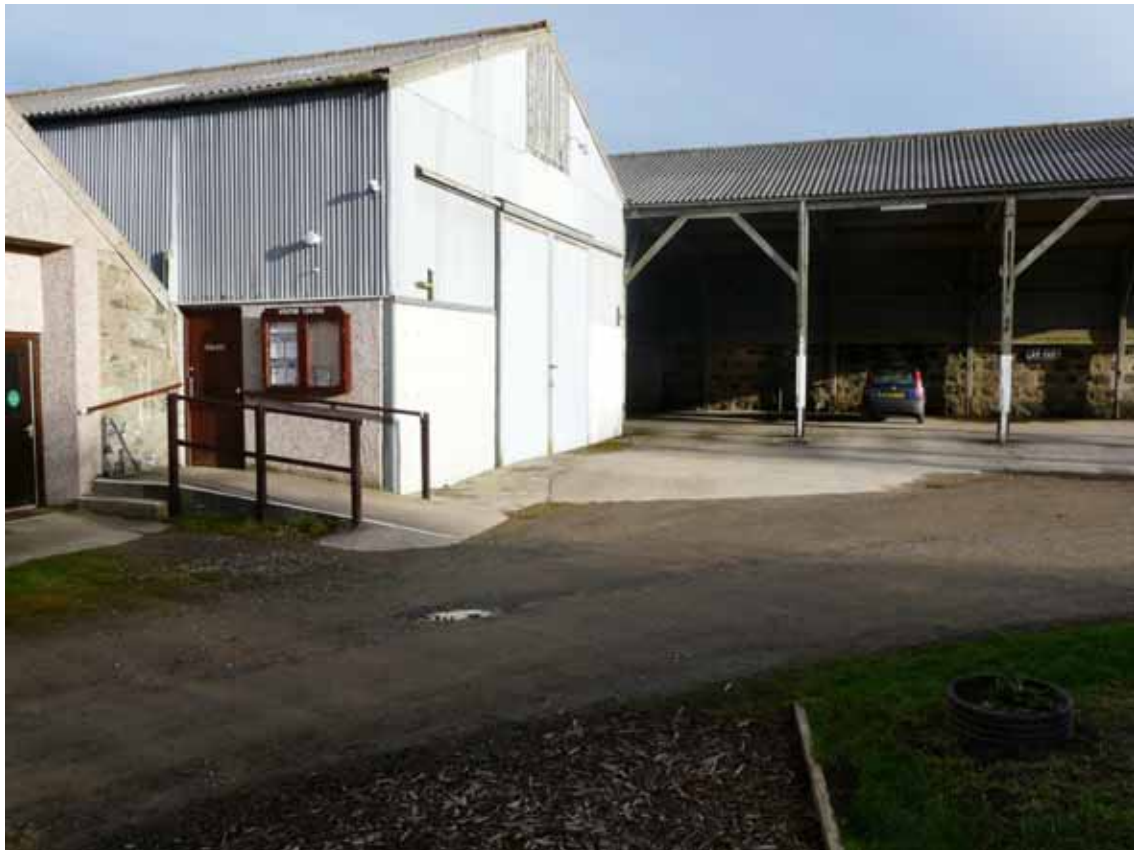
Car park with Visitor Centre and toilets on the left
